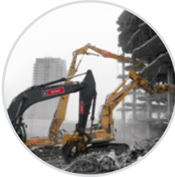
DEMOLITION & SITE CLEAN-UPS ↗
